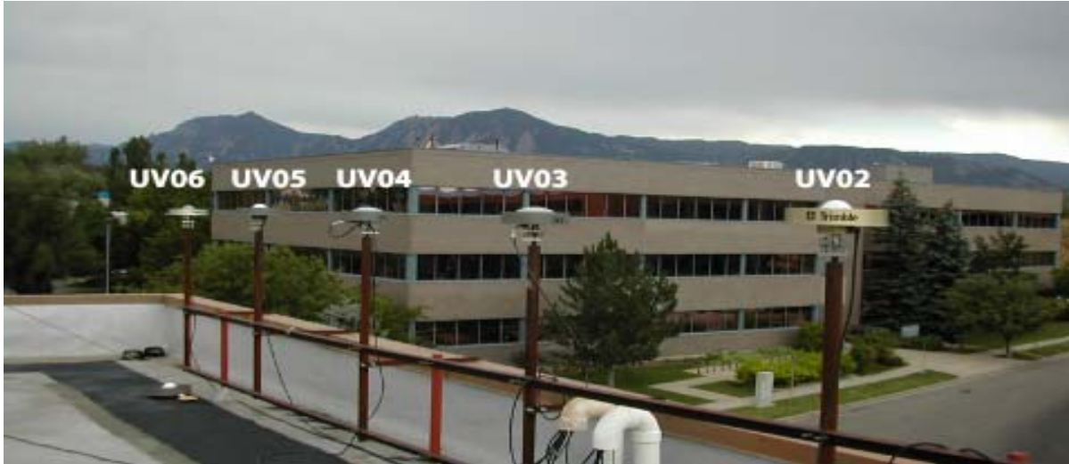
Figure 2.1 - Rooftop testing configuration looking southwest. UV06 is pictured at far left.
