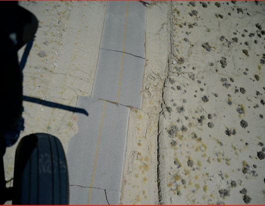
Fault offsets from the July 2019 Ridgecrest earthquakes.
