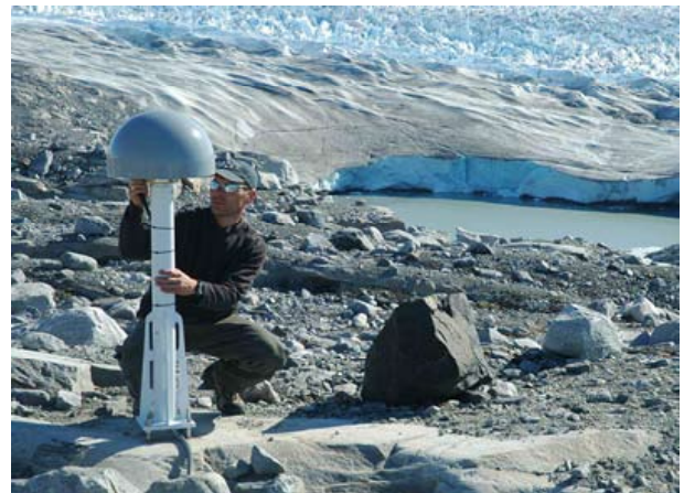
Figure 8 - Thomas Nysten of UNAVCO completes the antenna installation at GPS station KAGA above the Jakobshavn Gletscher/Kangia Icefjord.
