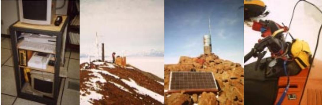
The differential corrections are generated at the MCM4 IGS site (at the NASA McMurdo Ground Station), with a receiver operating in parallel to the NASA continuously tracking TurboRogue receiver. The system transmitter is on Crater Hill, providing full coverage in the McMurdo Station vicinity and line of sight coverage throughout McMurdo Sound. A repeater provides coverage in Taylor Valley. The hand-held DGPS receivers are easily mounted on vehicles or hand carried as appropriate.
