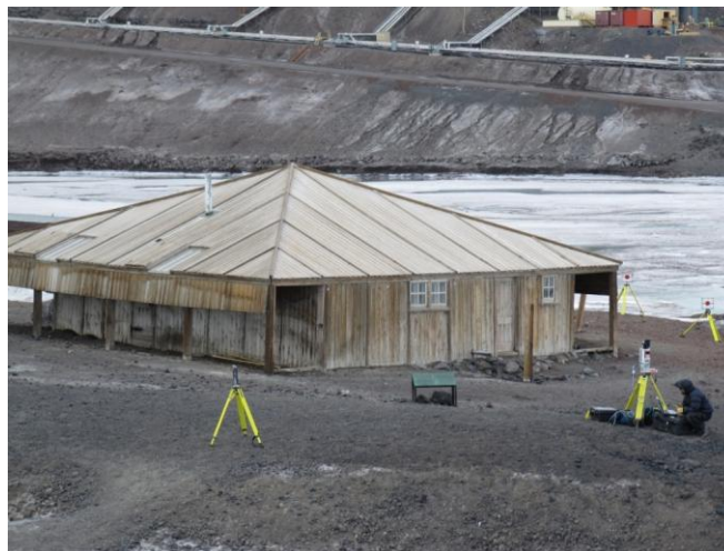
Figure 1: The Terrestrial Laser Scanner acquiring imagery at the Discovery Hut, McMurdo Station.
