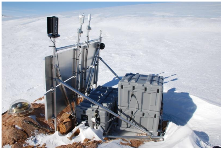
Figure 4: POLENET installation at the Clark Mountains, West Antarctica.
