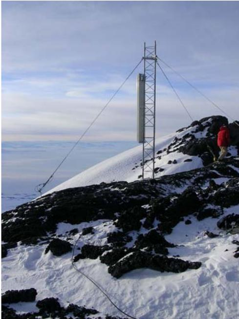
Figure 5a: Repeater tower at Truncated Cones. Note antenna on the left side of the tower.
