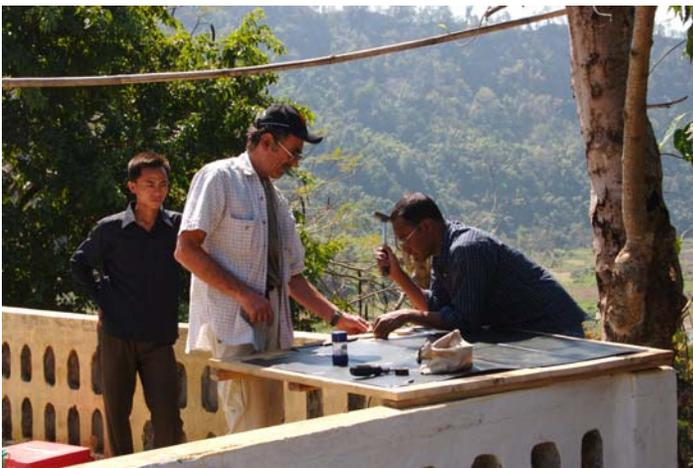
**Figure 3.** PI Leonardo Seeber of Lamont-Doherty Earth Observatory and Dhaka University student Dhiman Mondal construct the solar panel frame. GPS station BARK, the sole solar powered station in the network, is located at the Barkhol Upazilla (local government) officer's residence, on the east side of Lake Kaptai in the Chittagong Hill Tracts of southeast Bangladesh.
