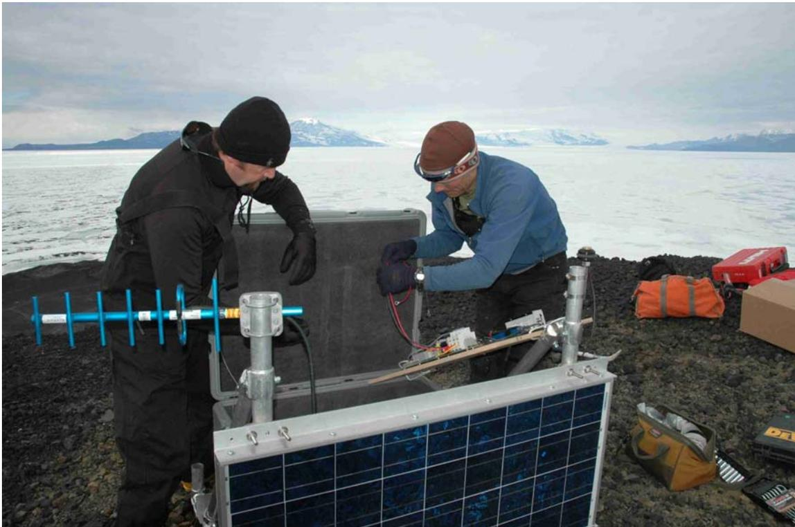
**Figure 7.** Raytheon Research Associate Jason Bryenton and UNAVCO field engineer Thomas Nylen set up a remotely operated RTK base station in support of the ANDRILL project.
