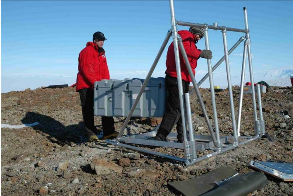
**Figure 8.** UNAVCO and PASSCAL MRI engineers Seth White and Tim Parker build the Minna Bluff extreme wind hardened GPS prototype at Minna Bluff, one of the windiest locations in Antarctica.
