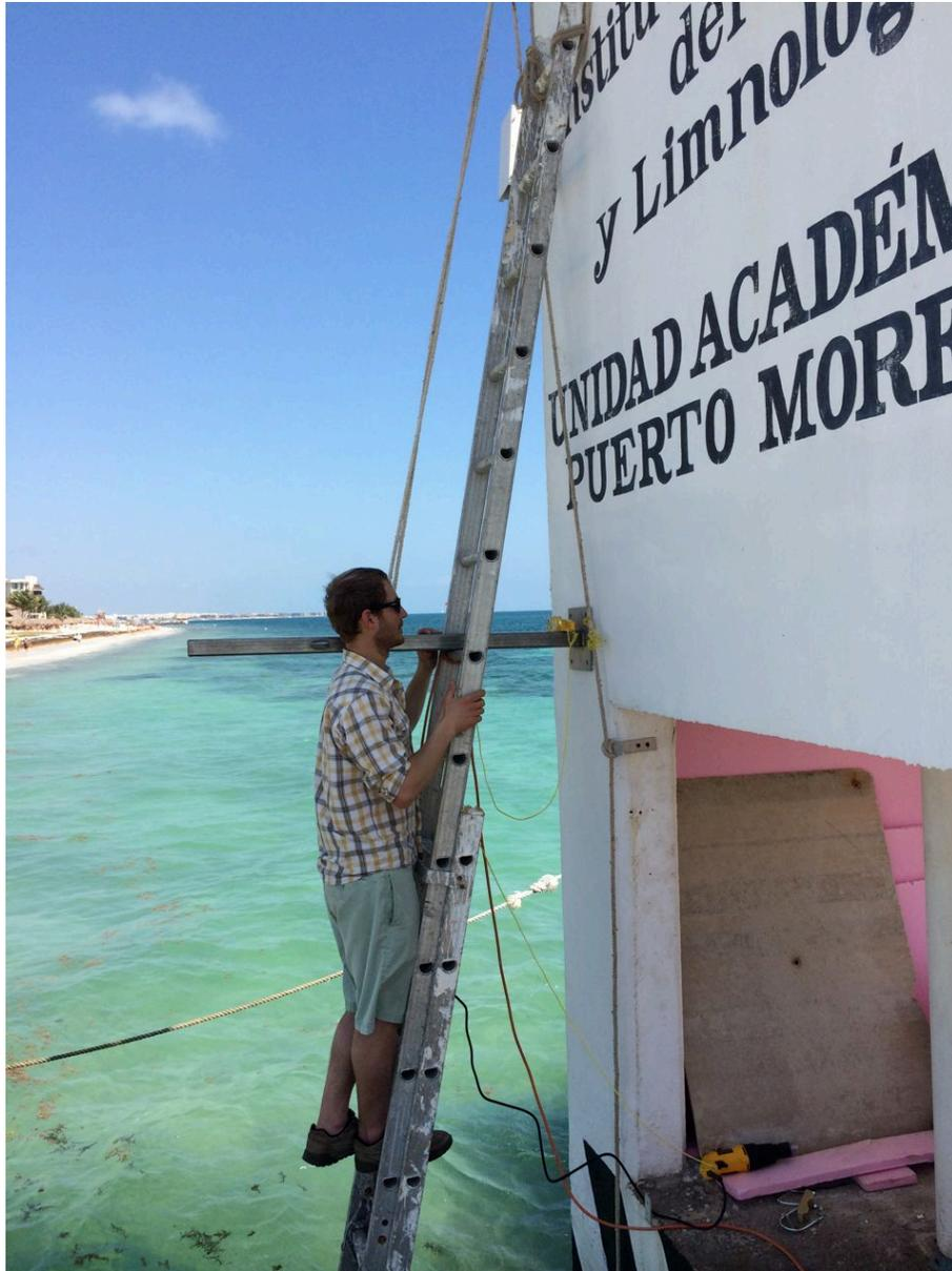
Figure 2. UNAVCO engineer Korey Dausz installing radar level recorder mount.
