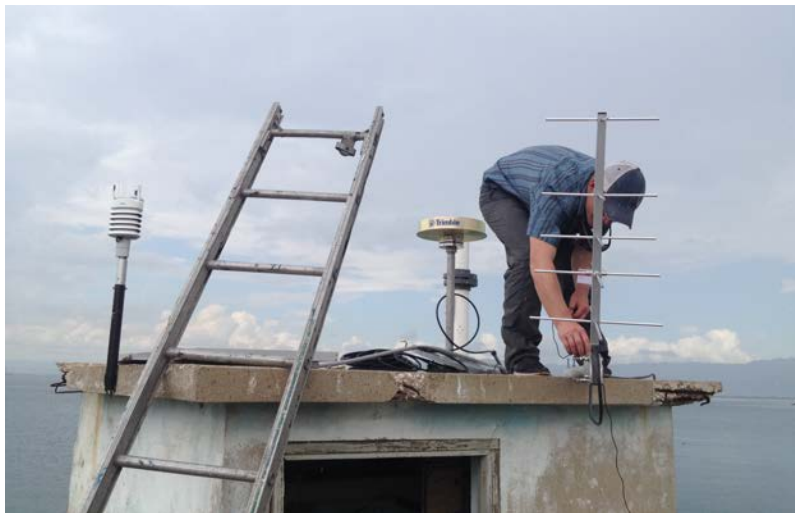
Figure 2: UNAVCO engineer Keith Williams installing the GOES satellite antenna.
