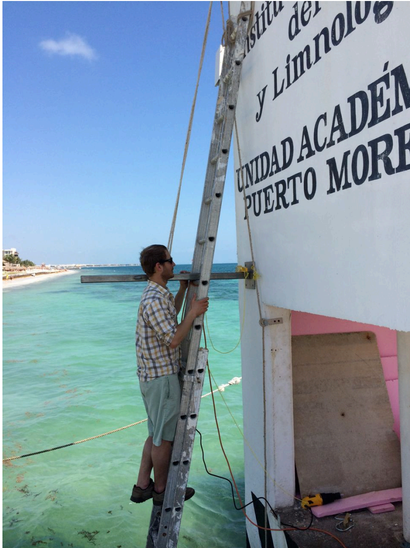
Figure 5. UNAVCO engineer Korey Dausz installing radar level recorder mount.
