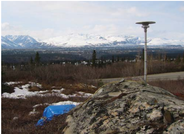
Figure 1. Photo of one of the continuous GPS sites, as installed after the earthquake. The monument was a 2-inch diameter invar rod, and the receiver and batteries were stored in a plastic tub wrapped in the blue tarp.
