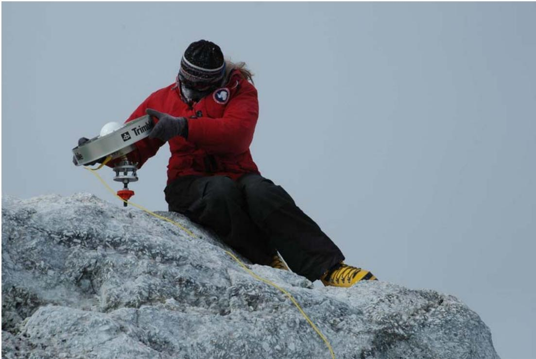
**Figure 1.** Project engineer Beth Bartel installing a GPS antenna on the rim of Mt. Erebus Volcano, Antarctica. Twenty-five individual projects were supported during the 2004-2005 Antarctic field season, which came to a successful close in March. More photographs of Erebus GPS monitoring can be found on the Erebus Volcano Observatory web site <http://www.ees.nmt.edu/Geop/mevo/mevomm/imagepages/gps/index.html>.
